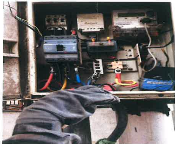
Hooking removal from Meter Pillar Box at Kamarhati
