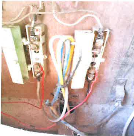
Hooking from service cut-out
