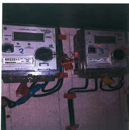
Meter tampered by making hole
